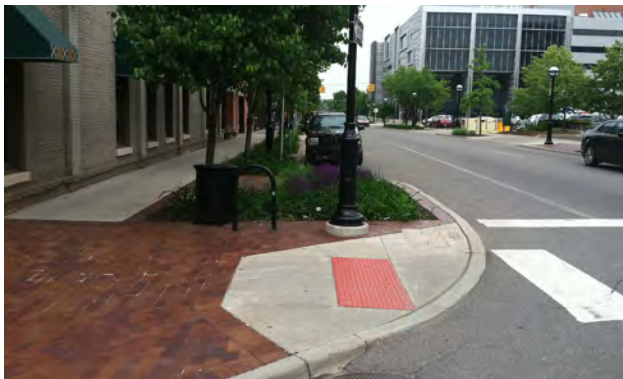
ADA compliant curb ramp
