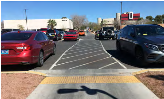
An ADA accessible path through a UNLV parking lot
