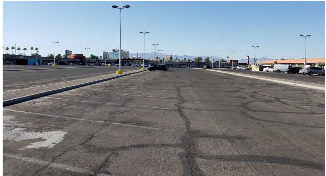
Lack of pedestrian connections through parking areas
