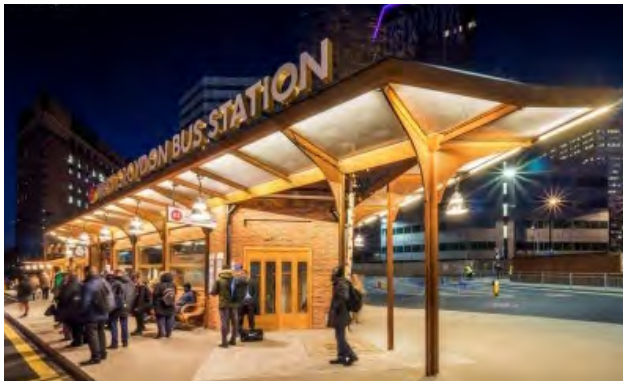
Well lit bus transfer station
