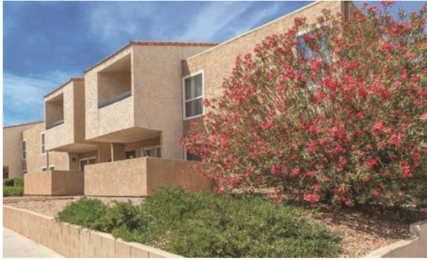
The Woodcreek apartments in Clark County serve residents who make 60% or less AMI. Private activity bonds will be used to renovate all 232 units. Image Credit: livewoodcreekapartments.com
