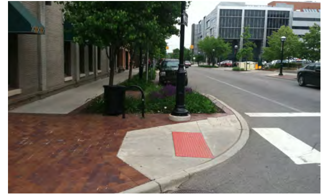
ADA compliant curb ramp
