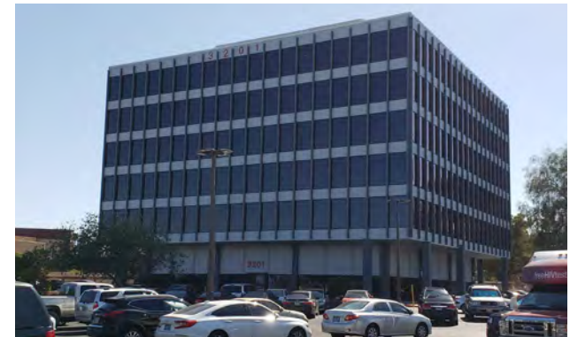
Medical offices west of Maryland Parkway
