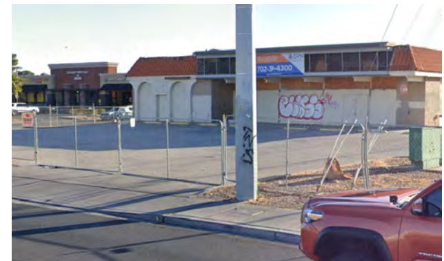
Lack of maintenance
