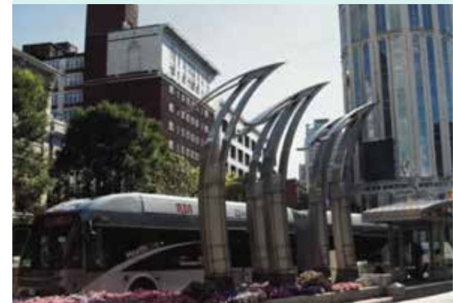
Figure 5: High-density development is seen behind a Health Line transit station along the Euclid Corridor in Cleveland, Ohio.
