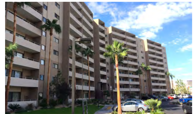
Multifamily high-rise along Flamingo Road
