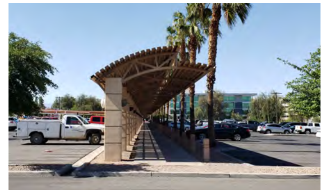
Covered pedestrian walkway near Sunrise Hospital
