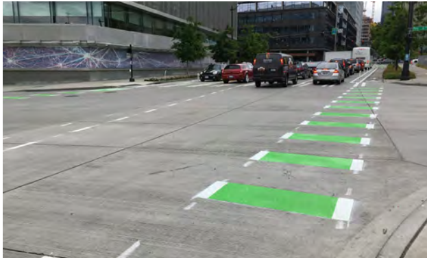
Bike crossing markings through an intersection
