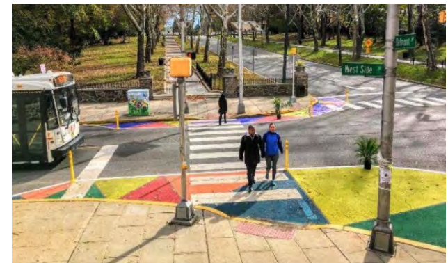
Temporary bulb out with paint and bollards
