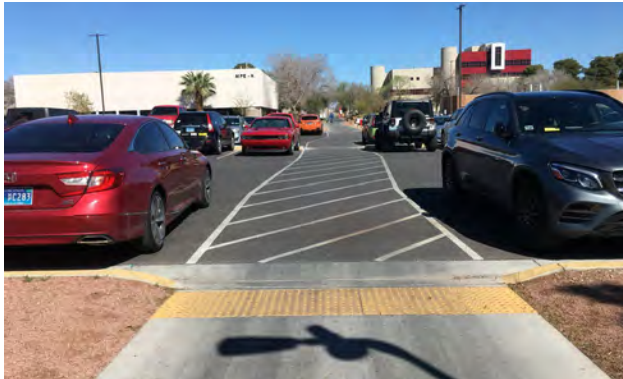
An accessible path through a parking lot at UNLV
