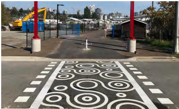
Thermoplastic paint in crosswalk
