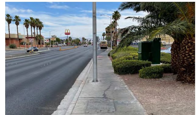
Sidewalk impeded by utility pole
