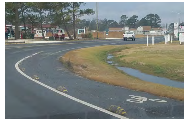
"Armadillos" help bike lane separation from traffic
