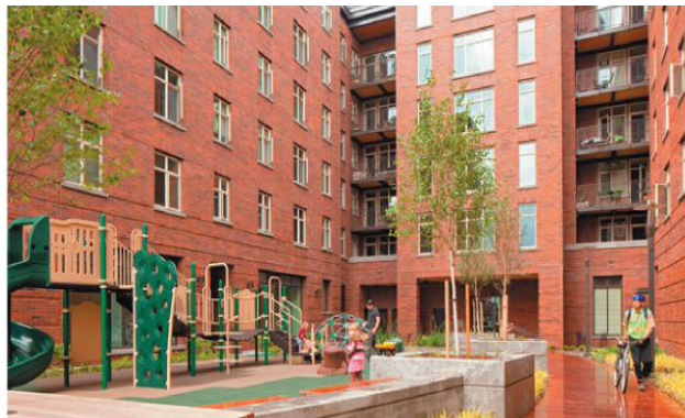
The Ramona Apartments, Portland
