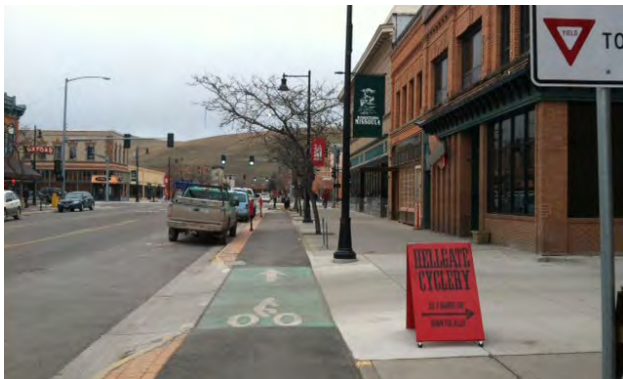
Driveway crossings should be clearly marked
